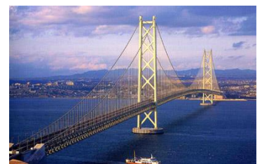
Akashi Kaikyo Bridge
